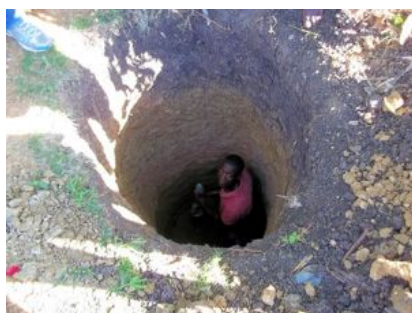
Digging Well by hand
