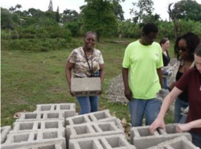
Lifting & carrying cinder blocks
